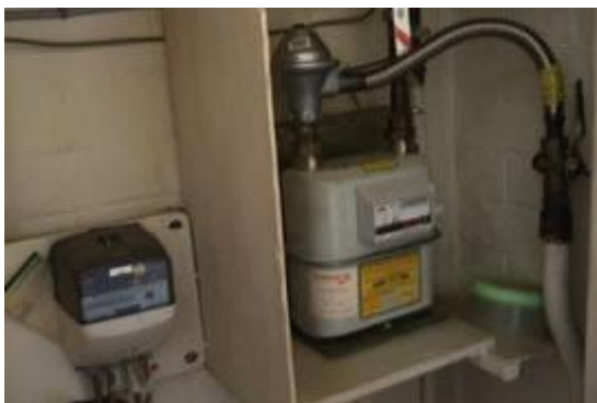
Asbestos panelling around a gas meter
