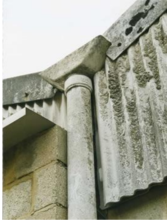
Asbestos cement downpipe, hopper and profile sheet
