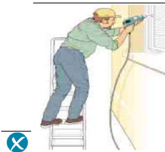
Incorrect – steps side on to work activity
