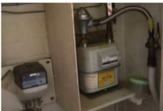
Asbestos panelling around a gas meter
