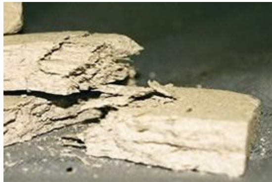
Pieces of Asbestos Insulating Board (AIB)
