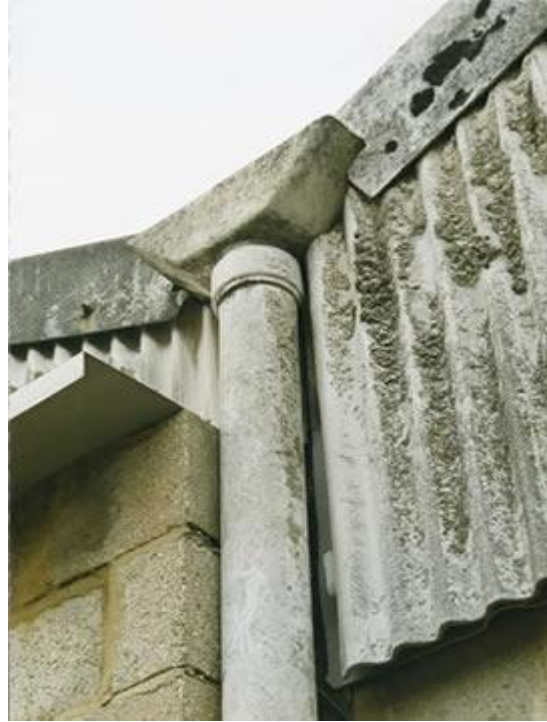
Asbestos cement downpipe, hopper and profile sheet
